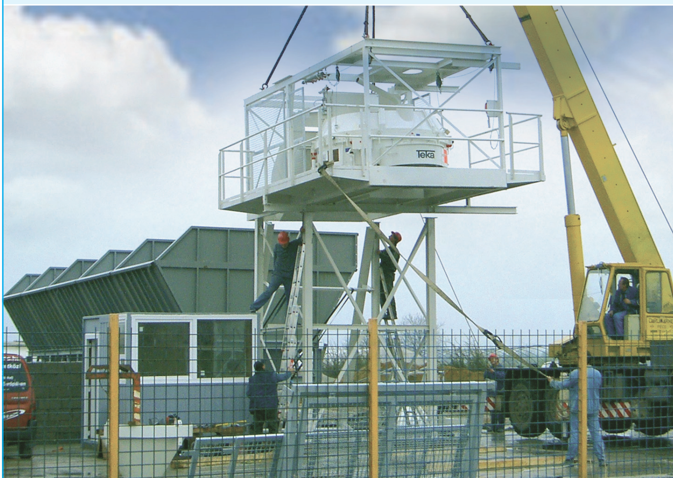
TRANSMIX THZ 1500 - R 5 Reihensiloanlage, 5 Kammern, Montage des Mischer-Moduls • TRANSMIX THZ 1500 - R 5 with aggregate in-line silo system, 5 compartments, erection of a mixer module
